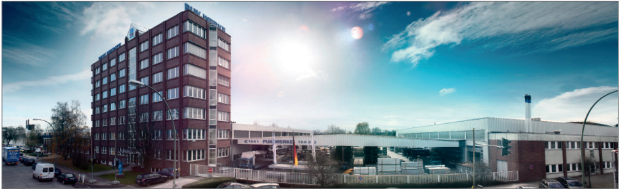
JORDAHL's registered office and administrative headquarters
