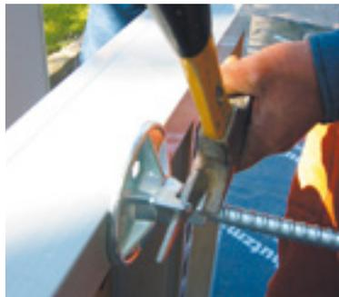
Set up the second formwork wall and tighten the formwork anchor.
