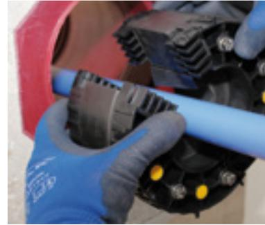
Fold the sealing element over the medium pipe and cable and push it all the way into the ribbed pipe. As an alternative to this, you can install both sealing elements from the inside. To do this, pinch off the stop lugs on the first sealing element and push it into the ribbed pipe. After this, proceed as described above.
