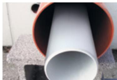
In the case of DN/OD 160 or 200 sewage pipes, use a DN/OD  $\geq 250$  settlement protection pipe; in the case of 250 mm medium pipe and cable, provide a settlement protection pipe  $\geq$  DN/OD 315; establish supports in the area of the outer basement wall.
