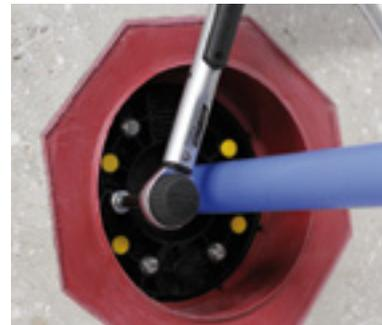
... use a torque wrench to tighten the screws to 6 Nm.
