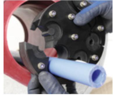
Fold the sealing element over the medium pipes and cables and push it to the stop edge into the ribbed pipe. As an alternative to this, you can push in both sealing elements from the inside.
