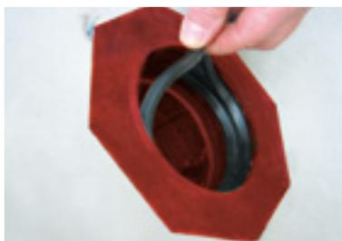
On the building side, insert lip sealing rings into the two beadings of the ribbed pipe.
