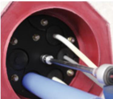
Tighten the screws in the diagonally opposite sequence in several passes. Start with the two screws in the middle. After this, use a torque wrench to tighten the screws to 6 Nm.
