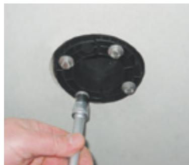
Tighten the screws in the diagonally opposite sequence in several passes with 6 Nm tightening torque.
