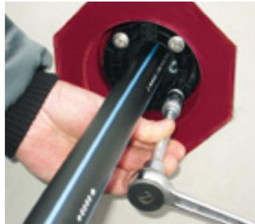
Tighten the screws in the diagonally opposite sequence in several passes. 6 Nm tightening torque.
