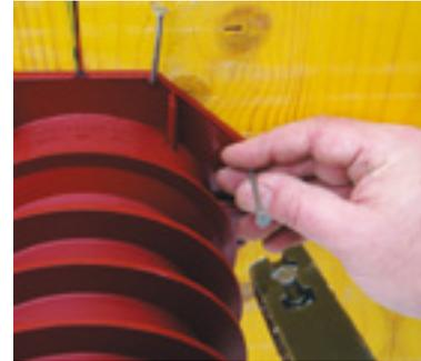
Nail the ribbed pipe to the formwork wall.
