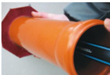
Insert the settlement protection pipe into the ribbed pipe.
