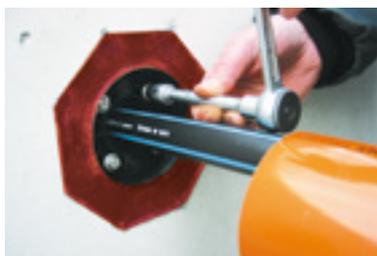
Tighten the screws in the diagonally opposite sequence in several passes with 6 Nm tightening torque.
