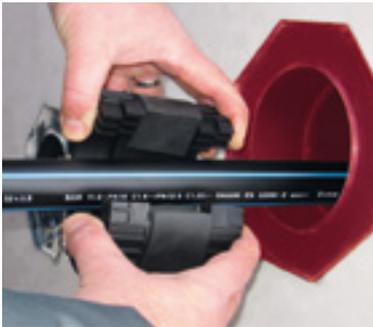
Fold the sealing element over the medium pipe and cable and push it all the way into the ribbed pipe. As an alternative, you can install both sealing elements from the inside. To do this, pinch off the stop lugs on the first sealing element and push it into the ribbed pipe.
