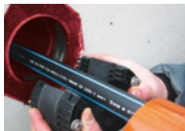
Fold the sealing element over the medium pipe and cable and push it all the way into the ribbed pipe.
