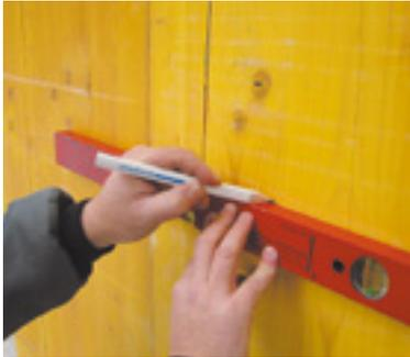
Mark the position of the pipe axis on the formwork wall.
