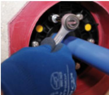
Tighten the screws in the diagonally opposite sequence in several passes. Start with the screws on the separation mechanism.
