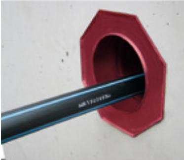
Push the medium pipe and cable through the concreted-in ribbed pipe.
