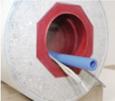
Push the medium pipes and cables through the concreted-in ribbed pipe.
